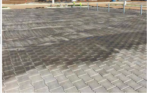
Close up immediately following sealant
