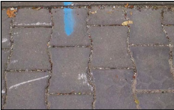
Photo 1 – PaveDrain in need of cleaning
