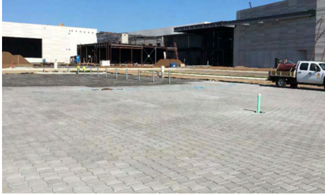
Sealant being applied on PaveDrain via Sprayer
