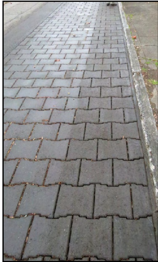
Figure: Bucher V-65 (top left), Elgin Whirlwind (bottom left), post cleaning (right). Any true vacuum, NOT regenerative vacuum would work.
