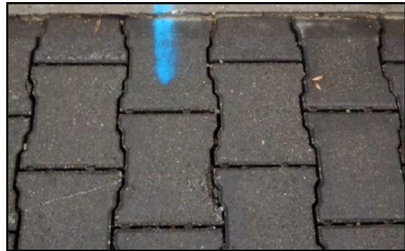
Photo 2 – PaveDrain following cleaning
