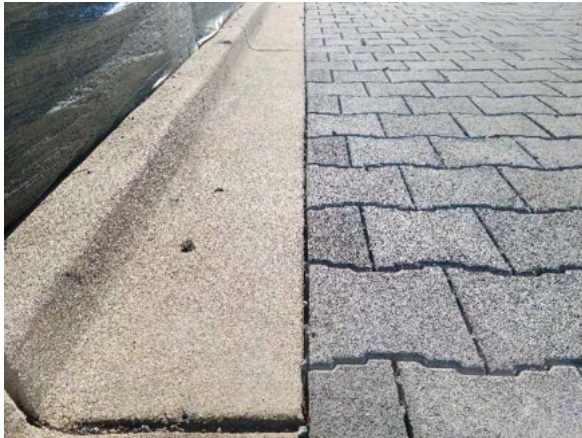
Pattern is designed to end in a clean edge with minimal cutting
