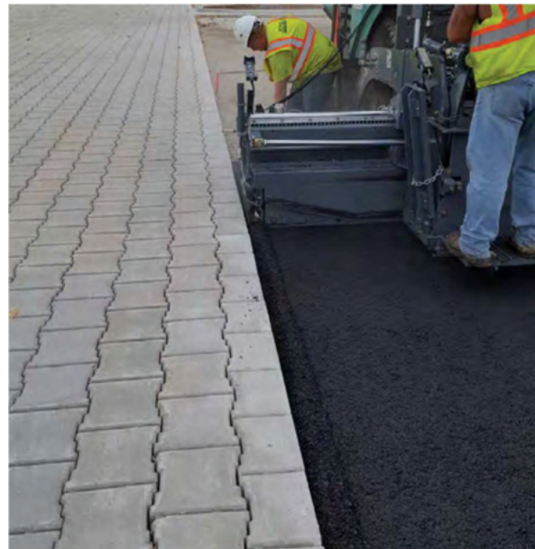
Pour the adjacent asphalt or concrete after placing the blocks
