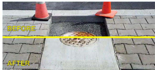
Square off manholes, observation ports, etc. with concrete collars
