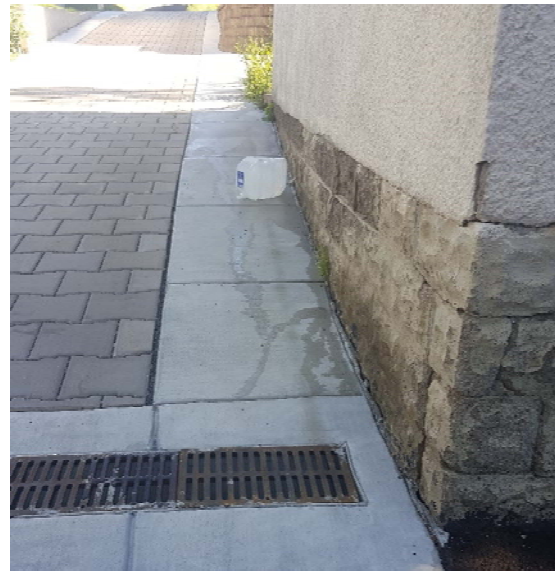
Field test showing runoff draining directly to the trench drain
