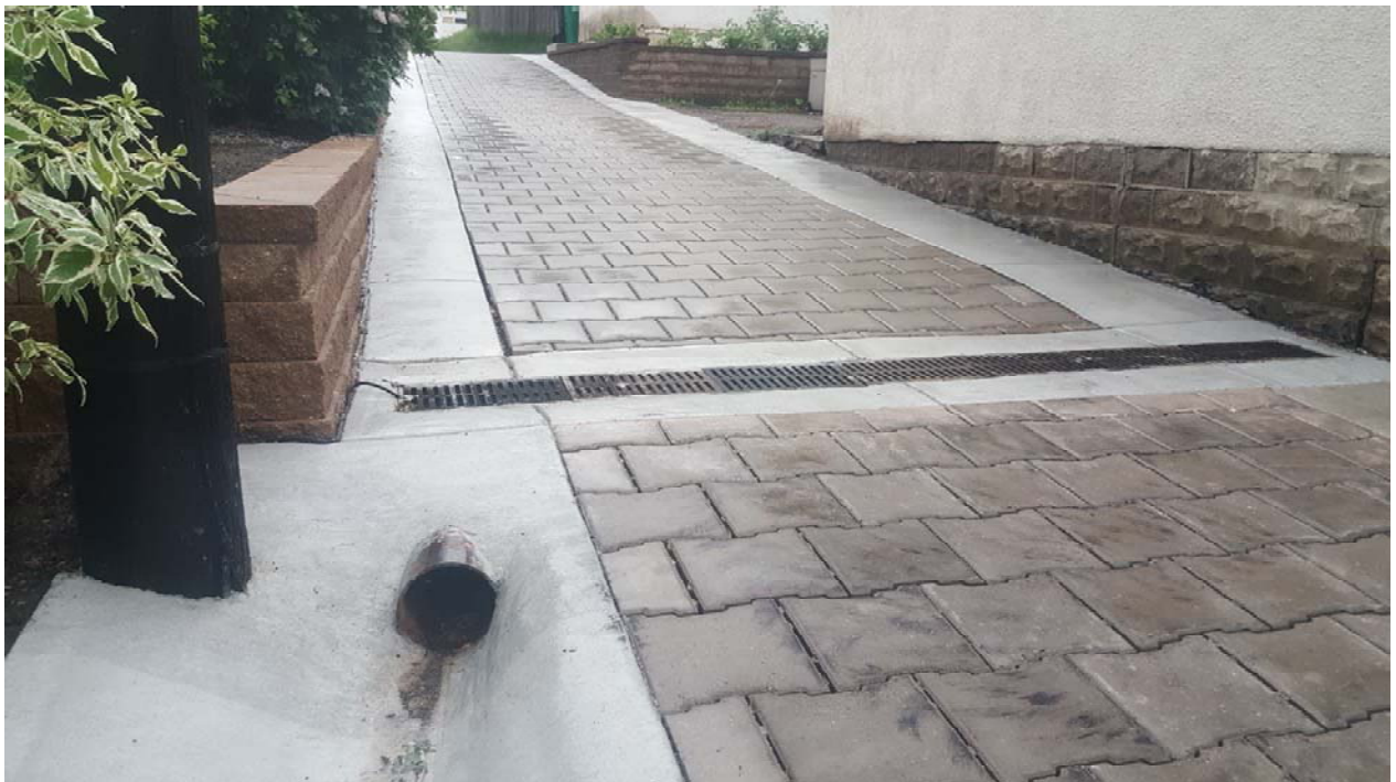
Complete PaveDrain alley, May 2018 Construction by JL Theis. Inc.
