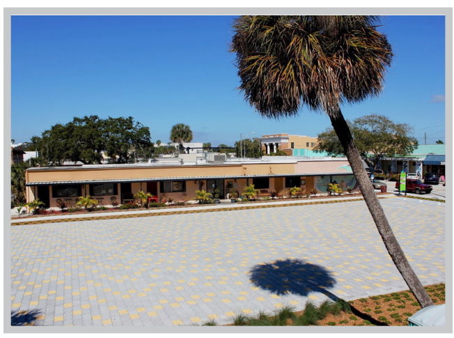
Completed job City of Melbourne
