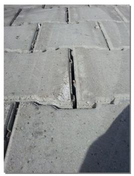
In order to minimize any surface damage to a PaveDrain block, the recommended snow plowing method would be with a rubber tipped snow blade. The following is an excerpt from a popular rubber snow blade provider. NOT AN ENDORSEMENT www.plowrubber.com
