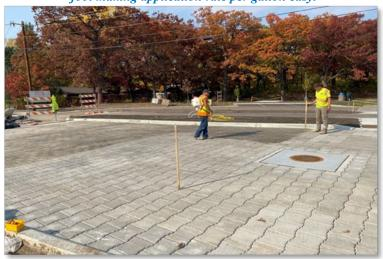
NOTE: It is strongly recommended to vacuum/clean the PaveDrain system prior to applying a sealant.
