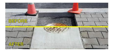
PaveDrain blocks work with existing infrastructure and can be used as the form for concrete or asphalt pours. Half blocks and end blocks square off corners eliminating cutting AND small pieces that are easier to dislodge.
